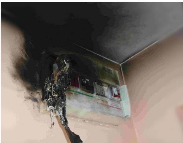
Result of a DIY home owner having wired an 10.5 kW electric shower circuit with 2.5 mm<sup>2</sup> cable and a 45 A circuit-breaker.
